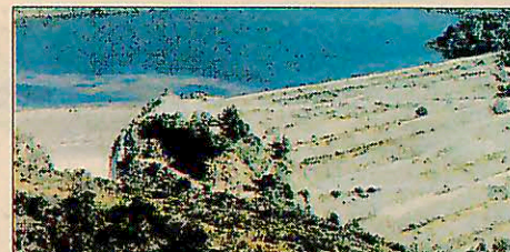
2 SAN GABRIEL DAM Purpose: Flood control & water conservation Type: Compacted earthfill and rockfill with concrete cutoff wall Elevation: 310 feet Construction began: 1932 Construction completed: 1939 Cost: $17 million
