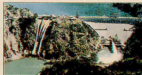
3 MORRIS DAM Purpose: Water conservation & flood control Type: Concrete gravity Elevation: 245 feet Construction began: 1932 Construction completed: 1935 Cost: $7.6 million
